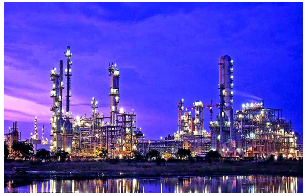
Aramco Jizan Refinery
