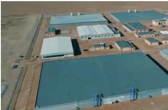
Al-Wajeeed strategic water filtration & treatment
