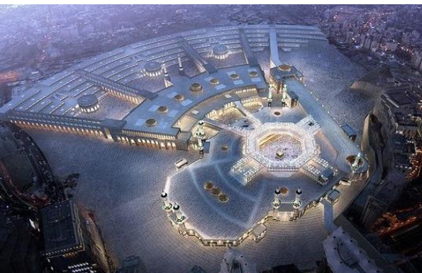
3rd Expansion of the Holy Haram Makkah & Surrounding Areas, Expansion Building, Piazza & Mataf
