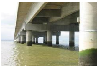
Concrete Repair & Protection Systems
