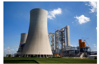
Power Generation Industry
