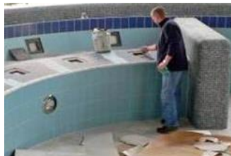
Tile Fixing Systems
